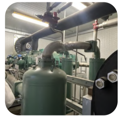
NH 3 refrigeration system - Plastuni Operations
