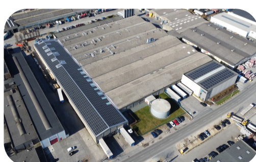
Solar panels - Plastuni Operations
