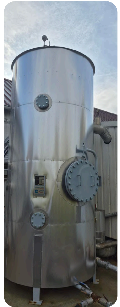
Water tank installed in 2025 Somater Mortagne
